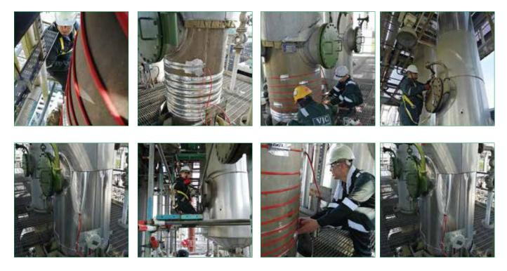
Installing New Heat Tracing Wire And Thermostat Enclosure, Testing & Commisioning
