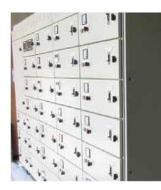
MCC stands for a motor control centre, MCC Control Panel consists of feeder for motor and blower and designed especially for motor operations. The MCC receives a signal from the control panel and which is used to control motor. The MCC is directly connected to the analogue motor. They are most commonly used in industrial and commercial facilities where there are plenty of electrical motors at use.
