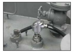
PT100 Sensor To Measure The Oil Temperature
