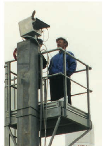
Linescanner in protective housing is mounted on top of a tower.
